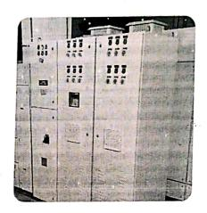
Function of APFC panel is improve the power factor. Most of the electric load is reactive, resulting in poor power factor. Companies distributing electricity encourage consumers to improve power factor. For improving power factor, electricity consumers have to connect
